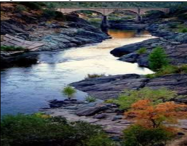
Fig. 5: Concrete bridge with its abutments on rocks 2 [22]
