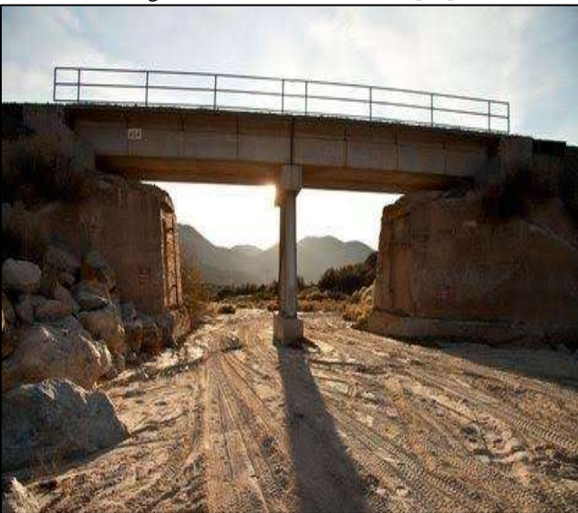
Fig. 4: Concrete bridge with its abutments on rocks 1 [21]
