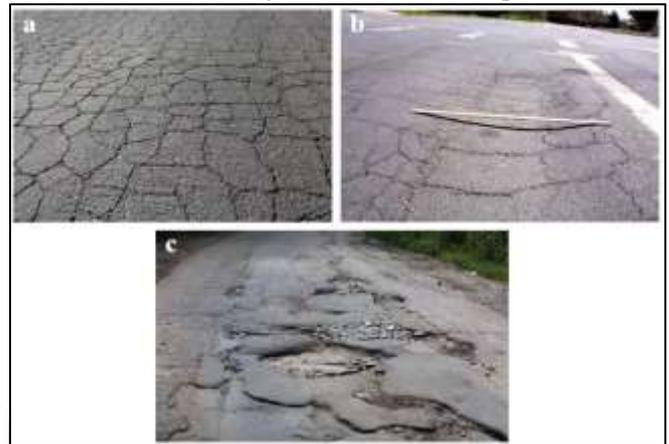
Fig. 1: Major failures in flexible pavements: (a) Fatigue cracking (b) Rutting (c) Pothole formation
