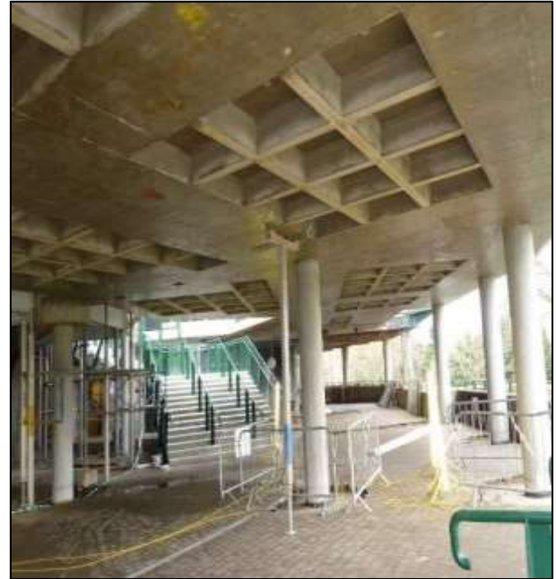
Fig. 2: One way and two way Ribbed Slab
