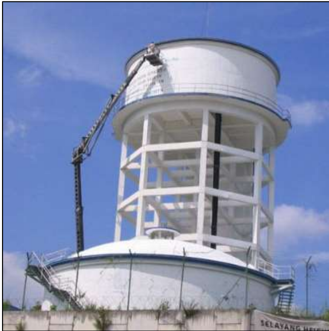
Fig. 1: Elevated water tank
