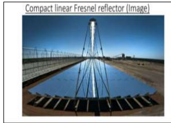
The constructional view of the Compact Linear Fresnel Reflector
