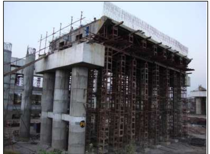
Reference Picture of Pier & Staging of Box Girder
