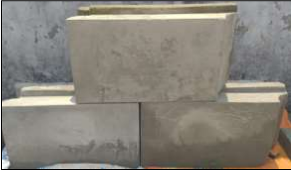
Fig. 2: (b) bond of interlocking Block.
