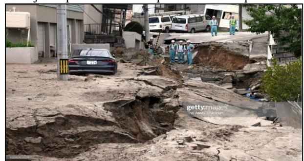
Fig. 1: Soil Liquefaction
