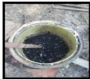
Fig. 4: Heat aggregate and Bitumen at 160°C
