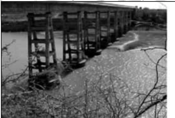
Fig. 3: The Rudramata Bridge, the tallest in the region, supported on open-type reinforced concrete A-frame piers.
