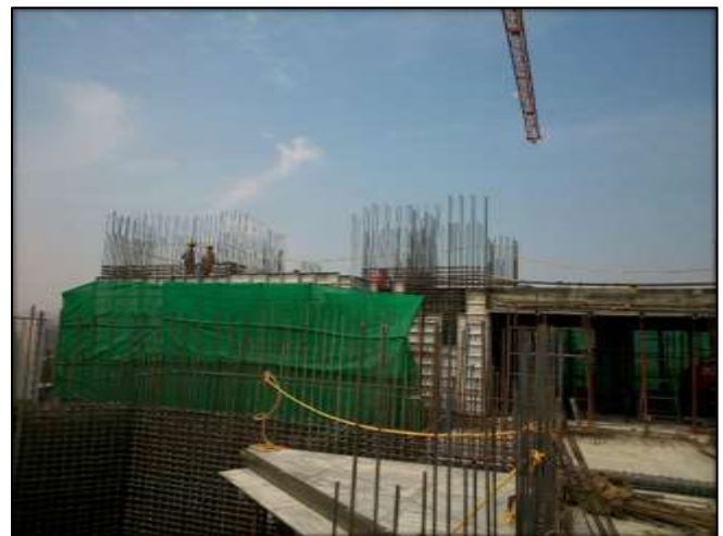
Fig. 1: Mulund construction site
