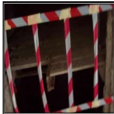
Fig. 5: Warning tape for an open hole.
