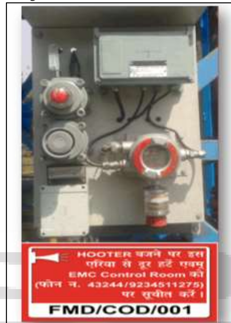
Fig. 1.0: CO Gas Detector in Tata Steel Works
