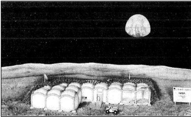
Fig. 3: Physical model of inflatable lunar base (Nowak et al. 1992)
