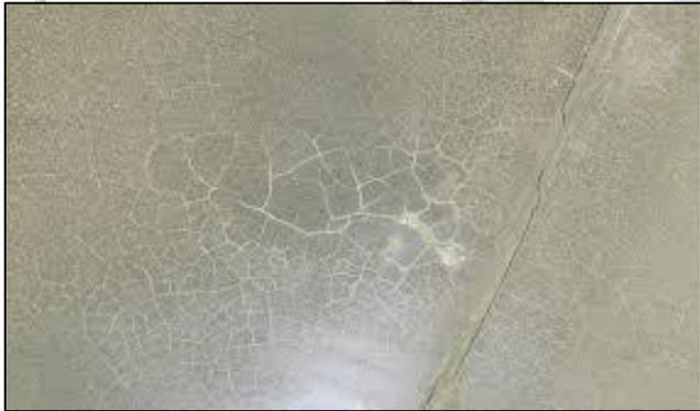
Fig. 4: Delamination of Concrete
