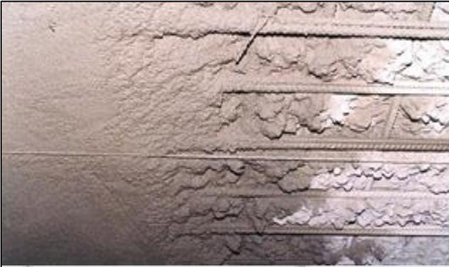
Fig. 2: Concreting of Fire Damaged Slab
