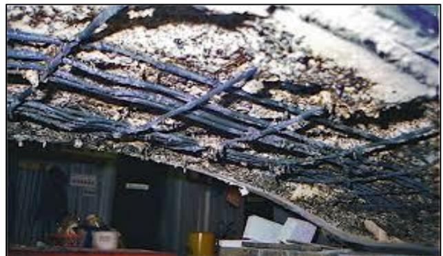
Fig. 3: Spalling of Concrete due to Fire
