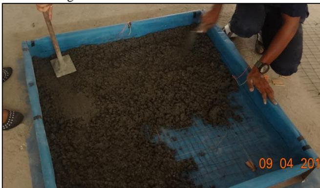
Fig. 5.1: Casting of conventional slab
