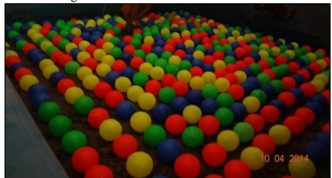
Fig. 5.2: Arrangements of plastic balls and casting of bubble deck slab
