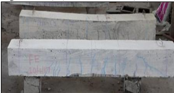
Fig. 10: Beam after Failure
