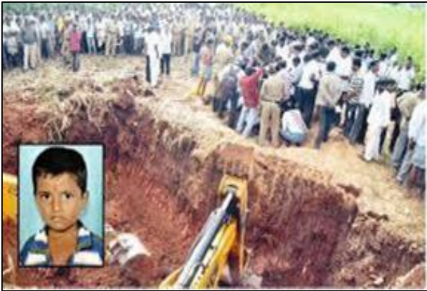
Fig. 1: Child rescuing from bore well by digging the parallel hole
