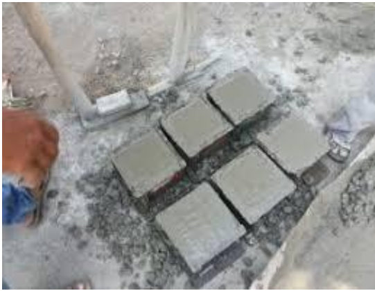
Fig. 2: Preparation of Moulds
