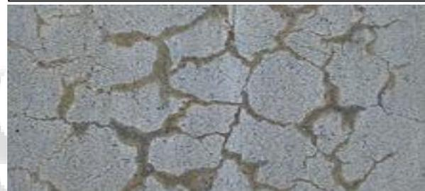
Typical crack pattern of the alkali-silica reaction (ASR). The gel exudations through the concrete cracks have a characteristic yellow color and a high pH.
