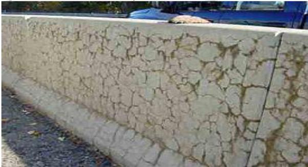
The alkali-silica reaction (ASR), more commonly known as "concrete cancer", is a swelling reaction that occurs over time in concrete between the highly alkaline cement paste and the reactive non-crystalline (amorphous) silica found in many common aggregates, given sufficient moisture.
