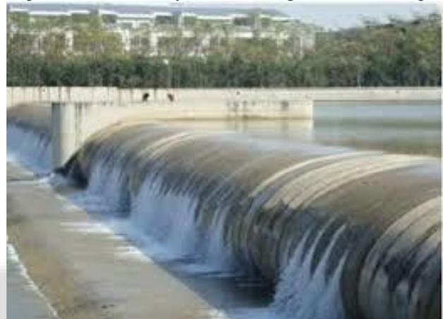
Fig. 1: Air filled rubber dam
