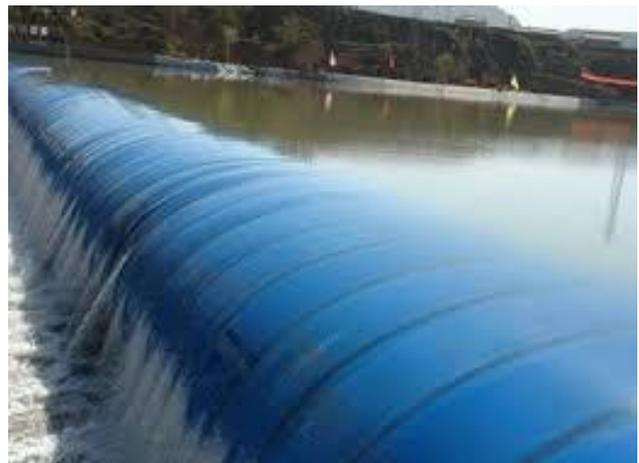
Fig. 1.2: water filled rubber dam
