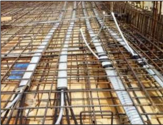
Fig. 2: Post Tensioning Slab
