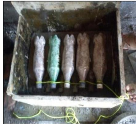
Fig. 4: Placing of Bottles and Mortar
