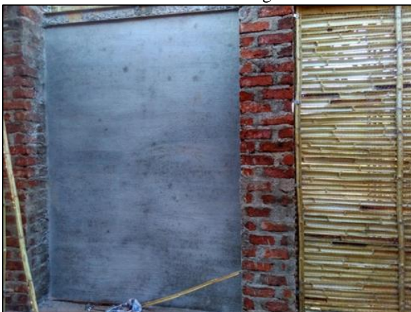
Fig. 2: Plastering of Wall Panel From Inside
