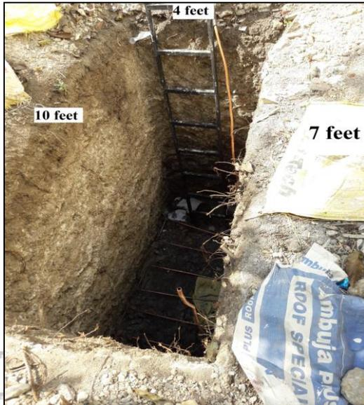
Fig. 6: Pit (Bore) for Copper EAHE
