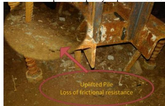
Fig. 5: Failure Due To Loss of Frictional Resistance
