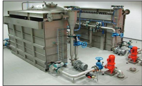
Fig. 2: Submerged Ultrafiltration Units
