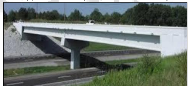
Fig. 1: High-performance concrete used in flyovers
