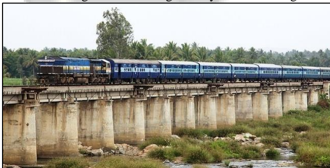
Fig. 1: Typical mass concrete solid gravity bridge piers [1]
