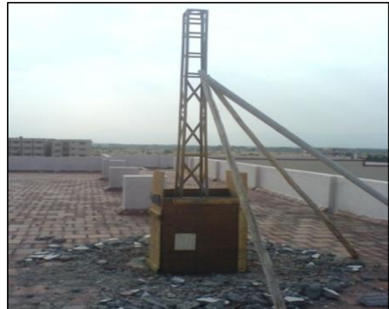
Fig. 5: Wind Mill Erection
