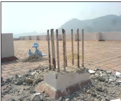
Fig. 4 : Wind Mill Foundation
