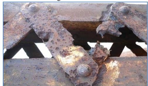
Fig. 3: Pitting corrosion
