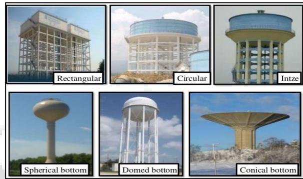
Fig. 1: R.C.C Storage Tank Types According To Shape
