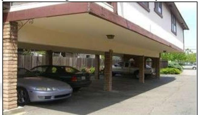
Fig. 1: Shows the soft story at ground floor, no infill walls are provided at ground story and fig. 2 shows soft stories at different floors used for office spaces
