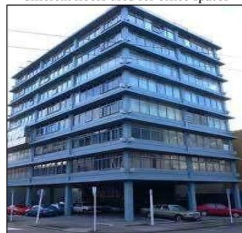
Fig. 2: Example of soft storey at different levels
