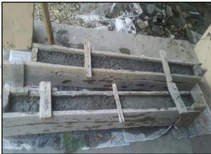
Fig. 3: Casting of Beams
