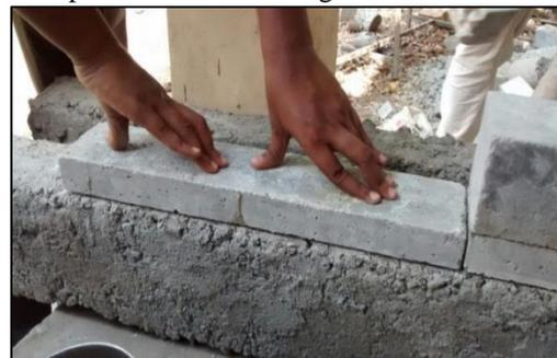
Fig. 6: Attaching Sifcon laminate over the beam surface
