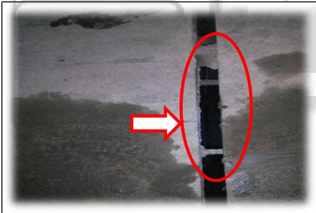
Fig. 2: Rigid Conduit through Slabs
