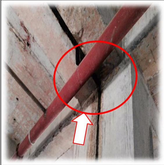
Fig. 10: Fire Fighting Rising Main at Expansion Joint
