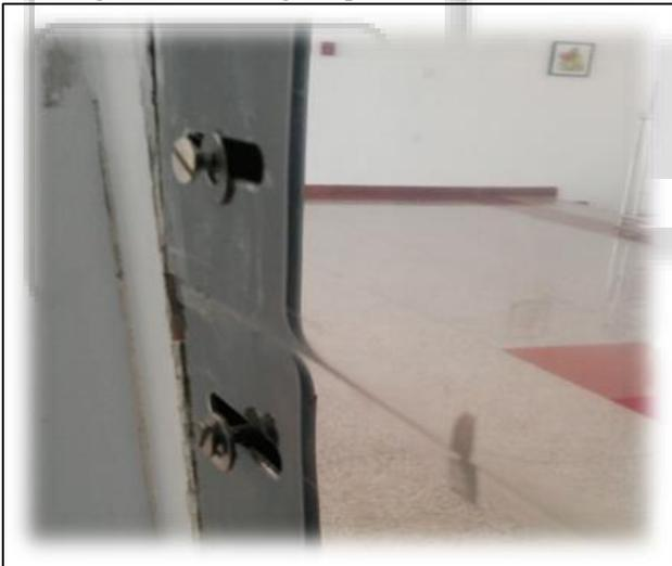
Fig. 16: Loosened Steel Screws
