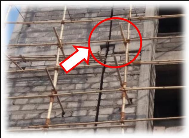
Fig. 15: Block work at Expansion Joint
