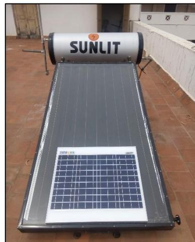
Fig. 11: Lower half covered PV/T Collector
