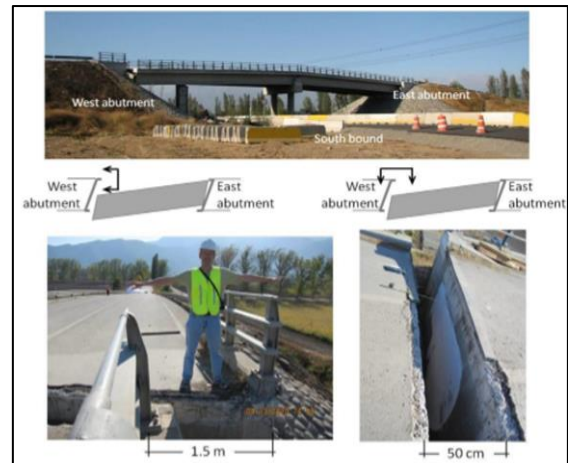
Fig. 2: Displacement and Rotation of Bridge
