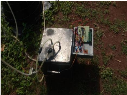
Fig. 4: Overall View of Thermal Storage Tank
