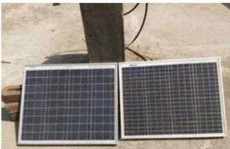
Fig. 6: polycrystalline solar panel
