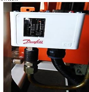
Fig. 14: Pressure switch
