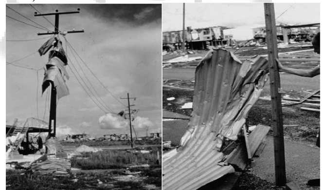
Fig. 1: (a) Catastrophic failure of metal (b) Cladding pulling over heads of roof cladding fasteners.
