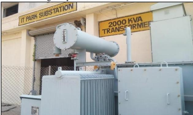
Fig. 1: 2000 KVA Step Down Transformer
