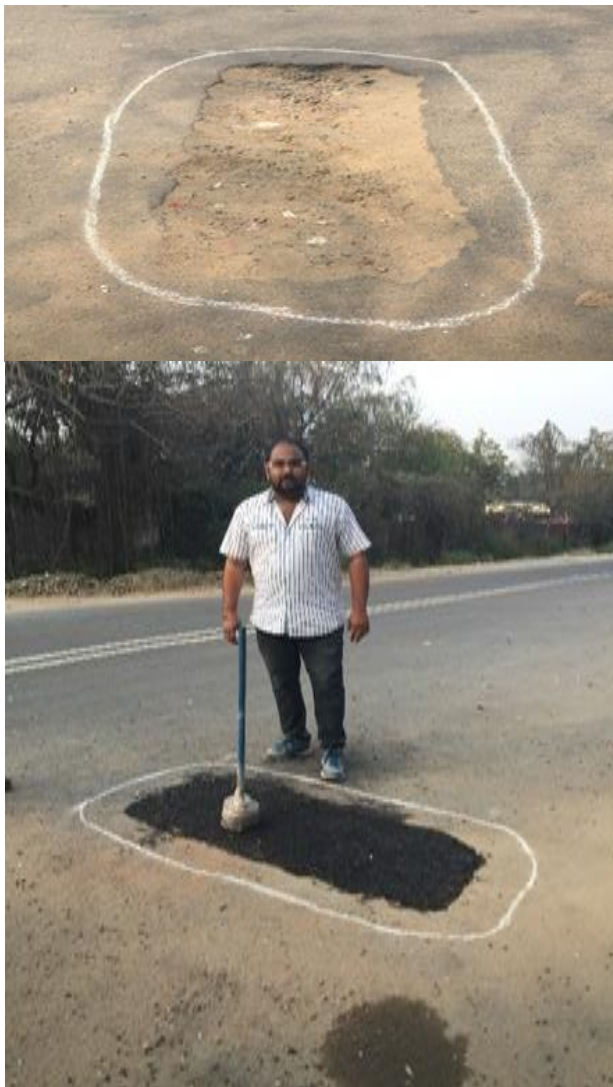
Fig. 6: potholes fill with natural aggregate and medium setting emulsion
