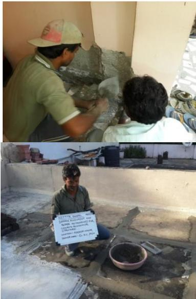
Fig. 3: Repairment by chicken mesh and major cracks filling
