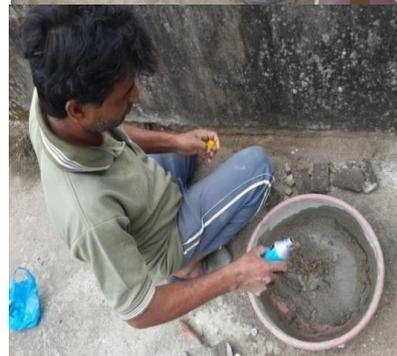
Fig. 2: Mortar preparation and adding Dr. Fixit in mixture
