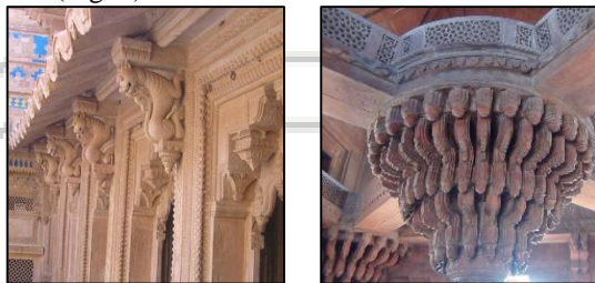
Fig. 1: Corbels are characteristic feature of Indian architecture
