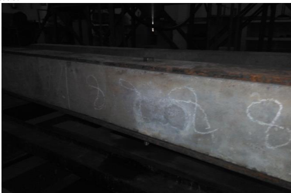
Fig. 3: Retrofitted with one plates top and one plate bottom of the beam
