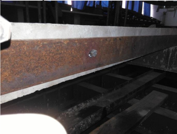
Fig. 7: Beam retrofitted with plates front and backside plate.
