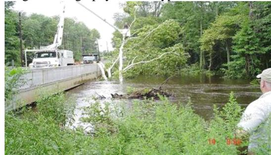
Fig. 7: Large Floating Debris Accumulation
