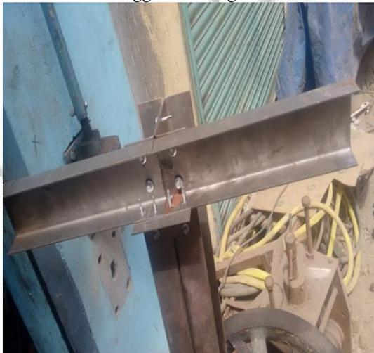
Fig. 2: Beam column connections using Self Tapered Screws in Linear arrangement of bolts
