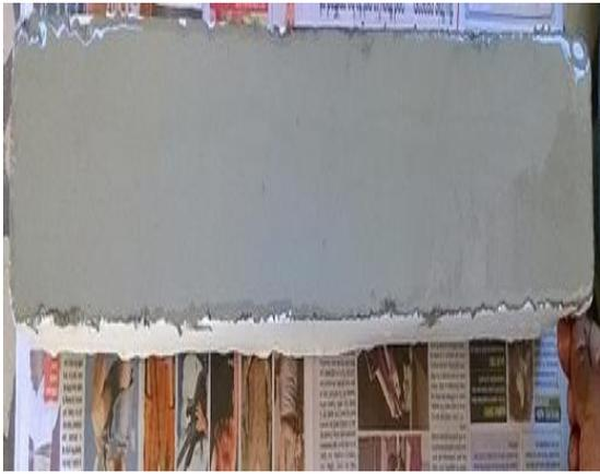
Fig. 4: Applying of Epoxy in the concrete beam
