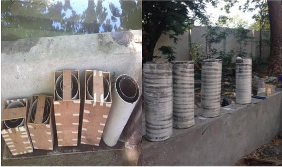
Fig. 4: Casting and forming of FRP tube
