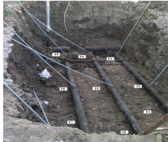
Fig. 5.1: Earth tube with sensors
