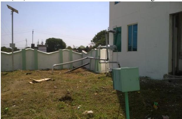
Fig. 5.1: Solar Photovoltaic Cell (PV) assisted Earth Air Tunnel Heat Exchanger
